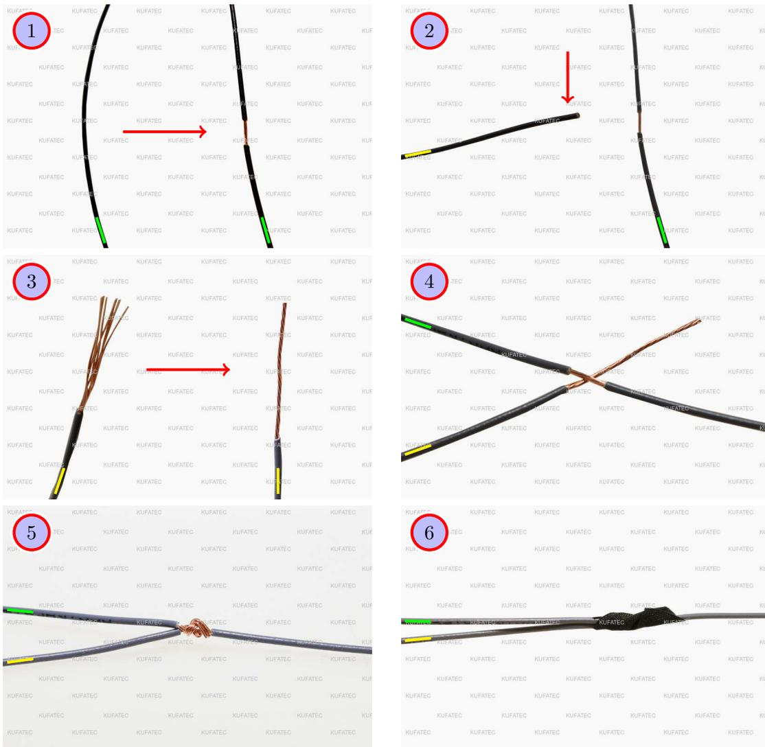
Figure 1: How to connect a cable to another
